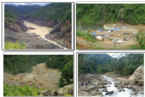
Figure 4. Debris flow Condition post crumbling natural dam.
